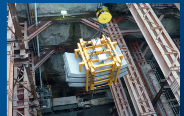
Self-powered hydraulic clamp
